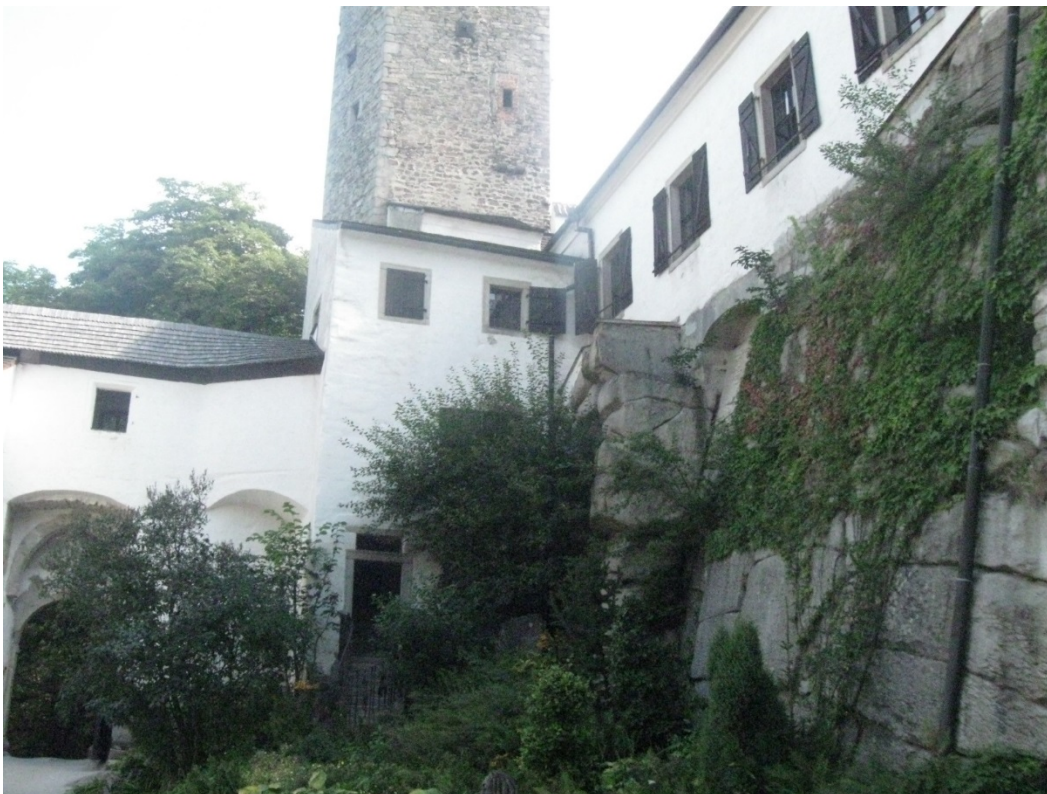
Fig. 2: Roštejn Castle: an example of incorporation of outcrops into buildings (Photo: Z. Máčka)
